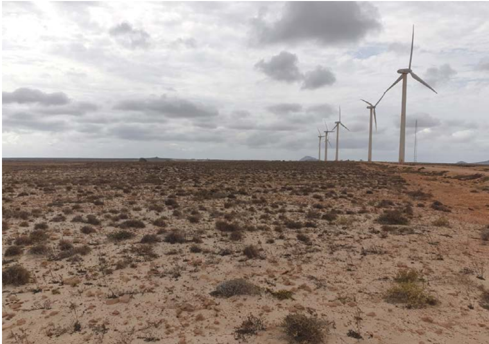
Figure 3: View of the south-eastern part of the wind farm territory, an area with high presence of the endemic and Critically Endangered Limonium brunneri .
